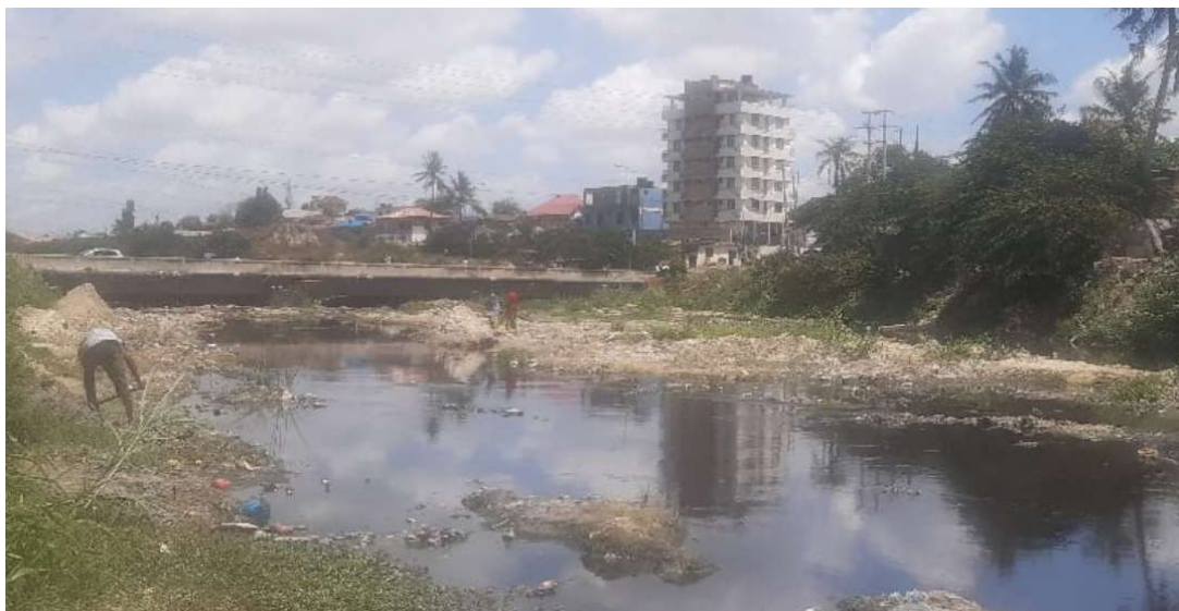
Picture 2-1: Narrow Water Passage & Accumulated Sand Resulting from River's Erosion Site Picture: August 2023
