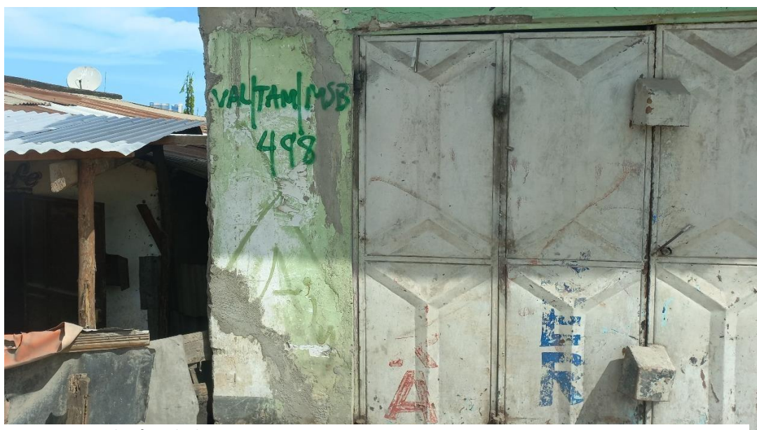
Figure 7-1: Example of marked structure
